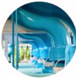
A/C COOLING WITH DSWC
